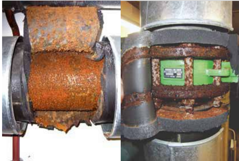
corroding steel pipes
