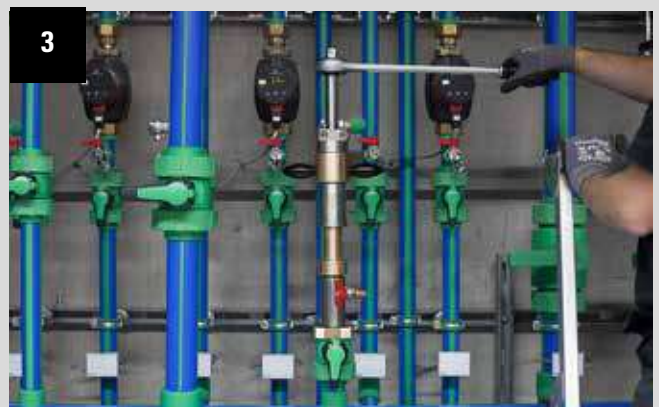
3. Start of the drilling process
