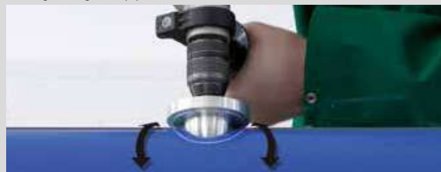
Removal of the oxygen barrier layer from the aquatherm blue pipe
