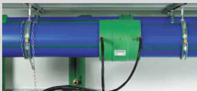
Adjust the socket diameter on the welding device. Start and control welding process. Keep the cooling time. Finished!
