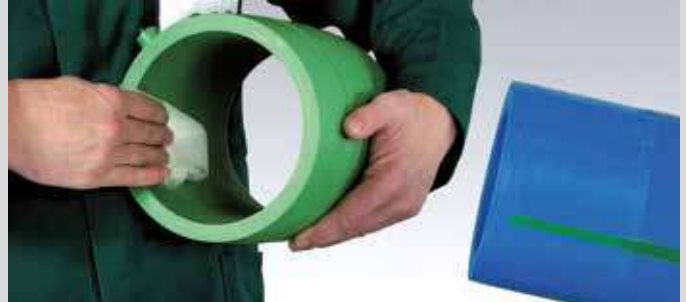
Clean the electrofusion socket's inner surface with a lint-free cloth or paper. Remove moisture that may occur immediately before the welding process again.
