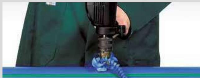
Drilling through the pipe wall
