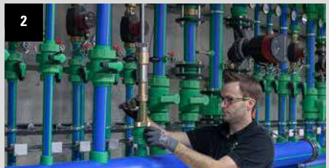
2. Assembly of the hot tapping tool onto the component
