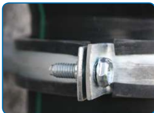
Figure 5 - Incorrect tightening:
