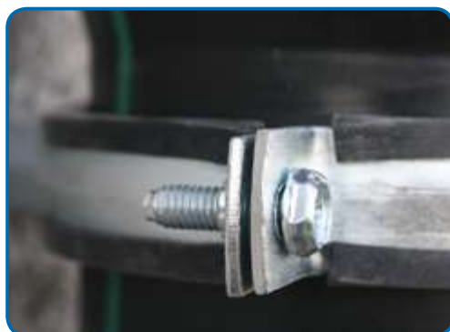
Figure 5 - Incorrect tightening:
